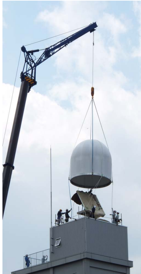
Installation of the Phased Array RADAR at the top of the building in Osaka University
